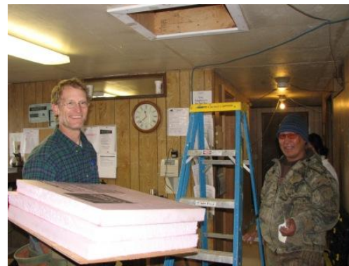
ABSN Project Manager Geoff Butler prepares rigid foam to insulate the City Office attic hatch cover
