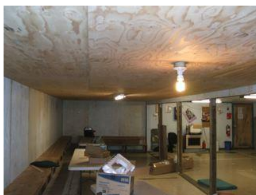
New plywood ceiling covering 2" rigid foam installed in 12' x 48' building addition
