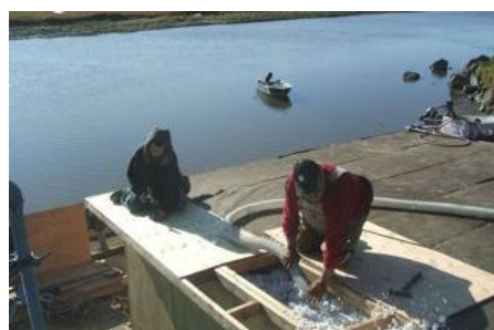
Local Wx workers add roof overhangs to the bldg perimeter – preparing for rigid foam installation on the exterior.
