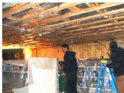
Local workers prepare ceiling for new plywood and air sealing
