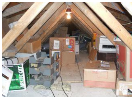
Nightmute Traditional Council Office attic pre weatherization – with many items stored in the attic compressing existing insulation
