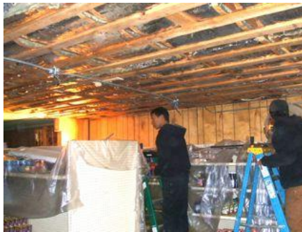
Local workers prepare the Chinuruk Store ceiling for new plywood and air sealing
