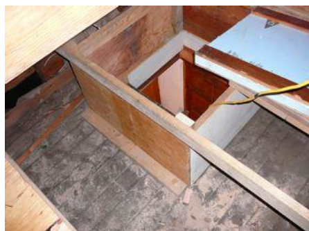
Attic with framed-in raised floor and attic hatch, ready for adding blown fiberglass insulation
