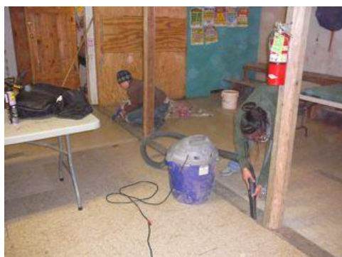
Anna Hilbruner and Genevieve Anthony air sealing where addition meets original bldg. Vacuum is used to clear debris before sealing
