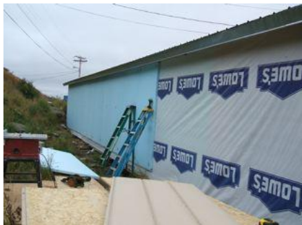
Chinuruk Store receives OIT, Outside Insulation Technique: 2" extruded polystyrene and new siding around full building exterior.
