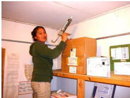
Local weatherization worker Genevieve Anthony air sealing in the City Post Office
