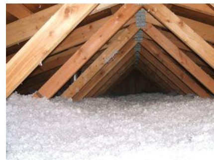
New blown-in attic insulation combines with existing reinstalled R19 fiberglass bats for a total of R49
