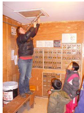
Anna Hilbruner air seals around the attic hatch cover.
