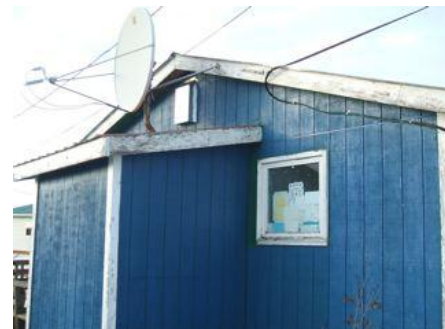
New gable-end vent with wind baffle cover installed on windward side of building.
