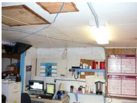
Two former furnace chimney / ceiling penetrations patched
