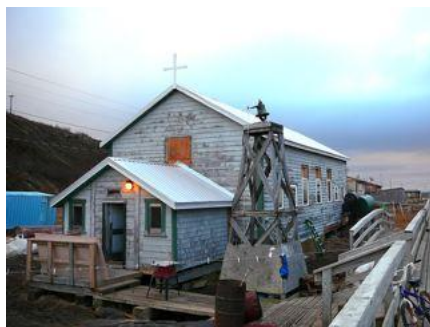
Community Church with new roof
