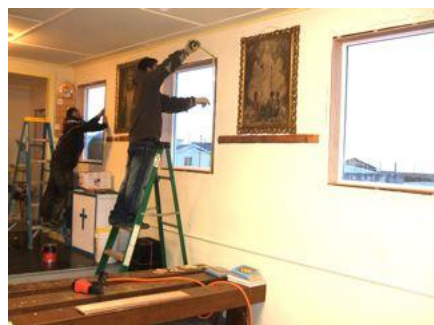
Local weatherization workers add trim to new triple-pane windows
