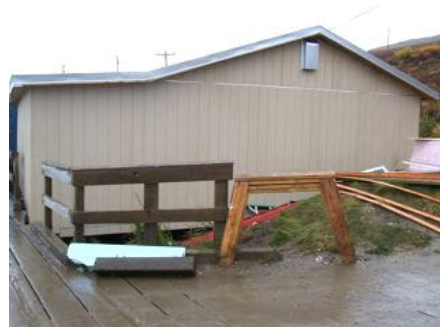
Completed store upgrades with new wind-baffle gable-end vent cover
