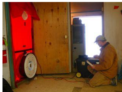
Geoff Butler sets up a blower-door test
