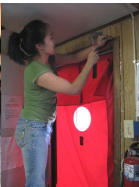
Local Weatherization worker Genevieve Anthony adjusts a blower door frame
