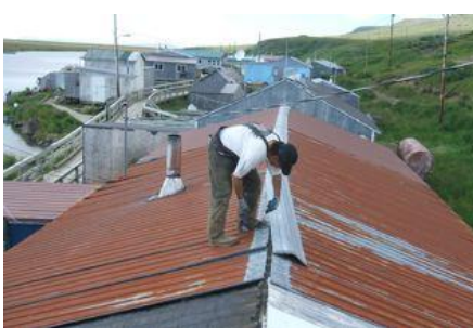
Local worker Joe Kosbruk removes old roofing panels
