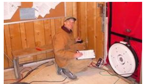
ABSN Project Manager Geoff Butler, starting a blower door air leakage test at the Nightmute Post Office
