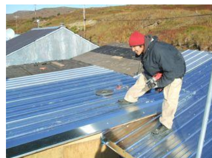
New galvanized metal roof in progress
