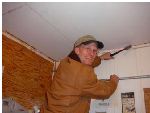
Tightening up cracks in wall – ceiling trim in preparation for air sealing
