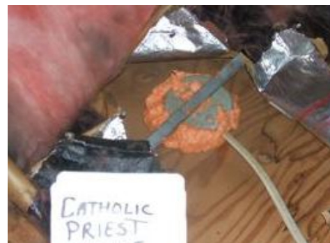
Foam air-sealing around a ceiling light fixture box
