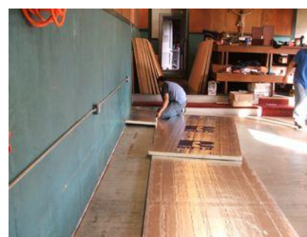
Local weatherization worker installs 2" rigid foam on main hall floor
