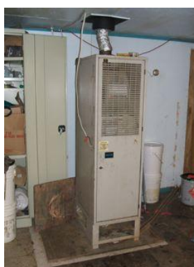
Old 70% forced-air furnace was removed and replaced
