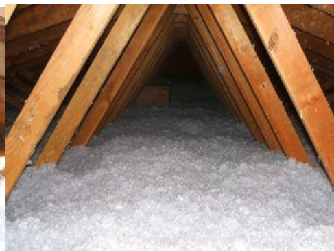
New blown-in fiberglass insulation to achieve total value of R42. After adding insulation Chinuruk requested permanently sealing attic hatch to prevent use as a storage area.
