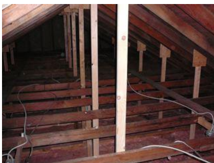
New framing to drop the ceiling 4' in preparation for adding R41 blown fiberglass
