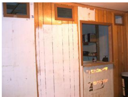
New passive air-flow vents (top) framed into wall to allow heat to disperse throughout the post office
