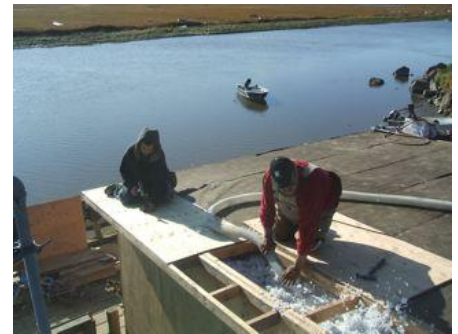
ABSN field manager Harry Morgan and Elliot Tulik adding roof overhang and blow-in insulation to the Chinuruk Store.
