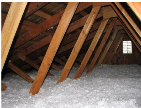
Blown fiberglass insulation on top of existing R19 fiberglass bats combine for an R47 ceiling
