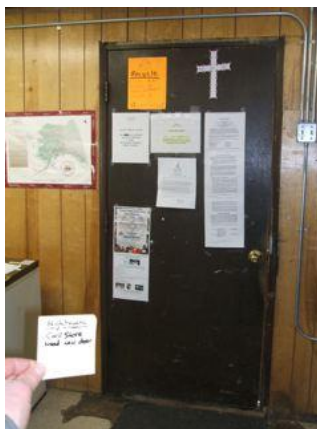
New insulated metal exterior door with weather stripping replaces old solid core door with no door jamb seal.
