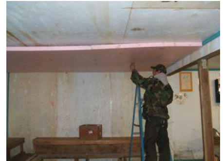
Installing 2" of rigid foam to ceiling of community bldg addition where roof is too low pitched for new blow-in insulation
