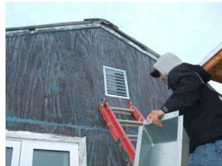
Local weatherization worker installing wind-baffle gable end vent cover
