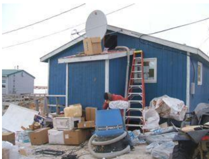
NTC Office during blow-fill insulation, with stored items from attic outside
