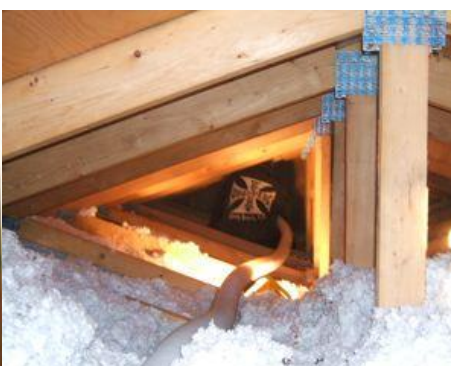
New blown-in fiberglass insulation to achieve total value of R42. After adding insulation Chinuruk requested permanently sealing attic hatch to prevent use as a storage area.
