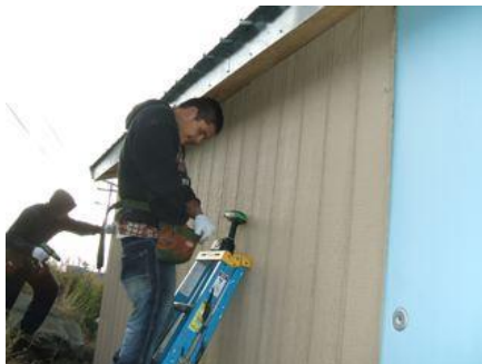
Chinuruk Store receives OIT, Outside Insulation Technique: 2" extruded polystyrene and new siding around full building exterior.
