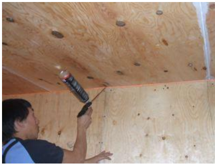
Air sealing cracks with spray foam
