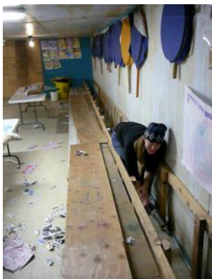
Plywood seating is removed and cracks are vacuumed before air sealing
