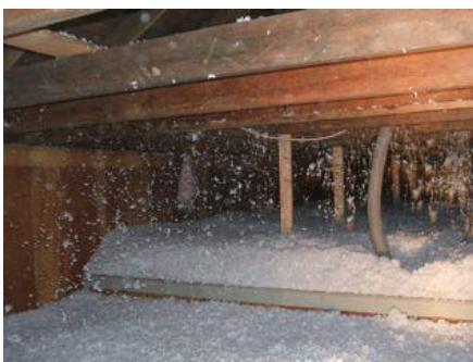
Blown fiberglass insulation going into new dropped ceiling area
