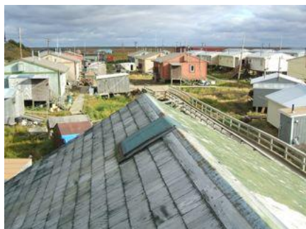
Old church roof – cedar shakes installed in 1947
