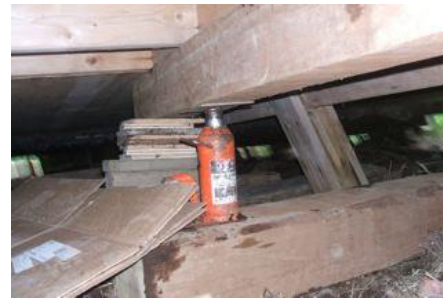
Extensive foundation jacking and leveling was necessary before energy measures could take place
