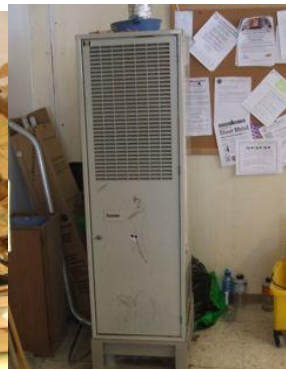
Old Miller forced-air furnace – discontinued as part of weatherization measures
