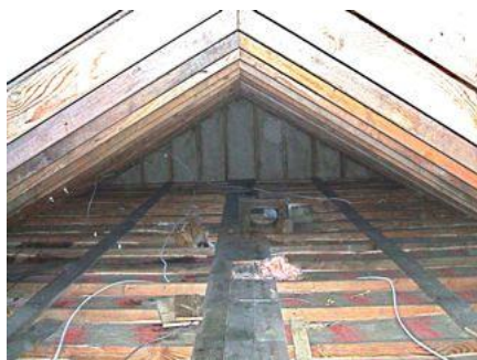
Former attic insulation: 1.5 inches: R4 fiberglass
