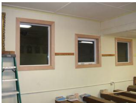
Completed new window installation
