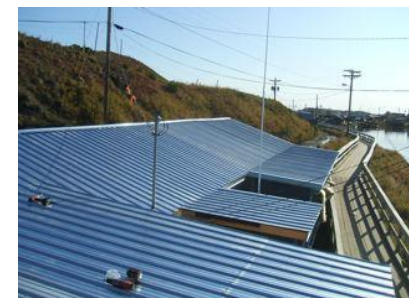
Local Wx workers add roof overhangs to the bldg perimeter – preparing for rigid foam installation on the exterior.
