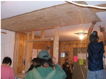
Installing new plywood over former forced air chimney penetration and water-damaged plywood
