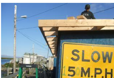
Local Wx workers add roof overhangs to the bldg perimeter – preparing for rigid foam installation on the exterior.
