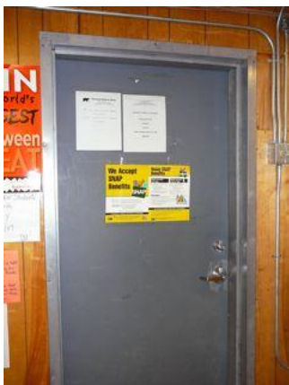
New insulated metal exterior door with weather stripping replaces old solid core door with no door jamb seal.
