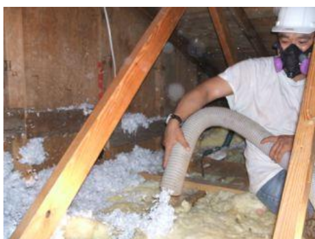
Adding blow-in fiberglass insulation
